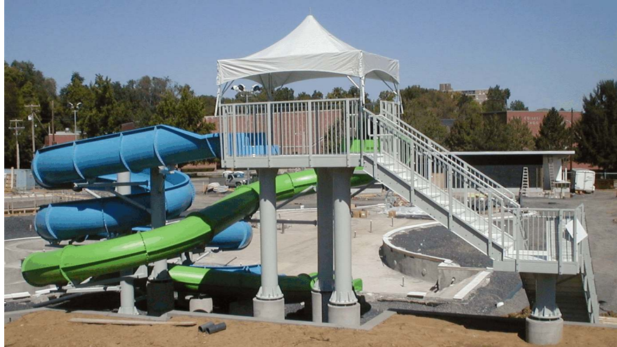
The new waterslides at Welch Pool (under construction).
